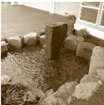
Above top to bottom: One of the team drilling a bronze basalt column using a 30 lb. pneumatic drill. Completed center stone feature with top of stone honed to disburse water evenly to all sides.
